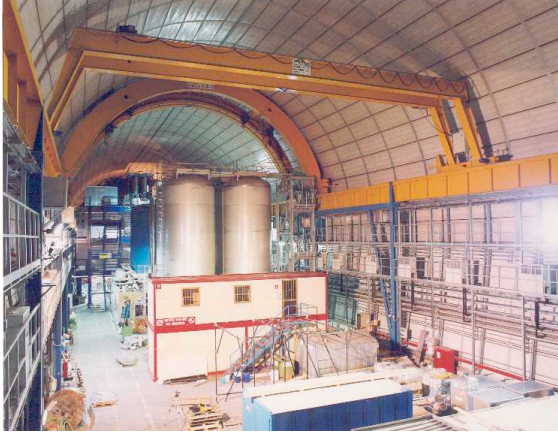
Figure 4. Hall C at LNGS, Italy. The hall is excavated in dolomite and is 20x20x100 m.
